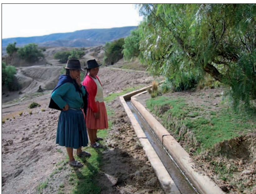
Figure 19 An irrigation channel in Bolivia
